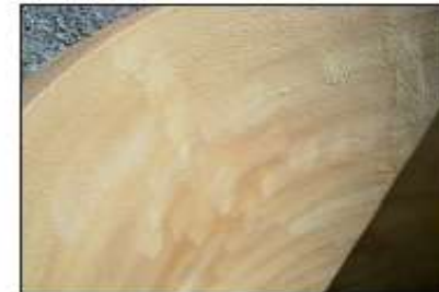
▲ Spraying Complete Collar ready for Installation
