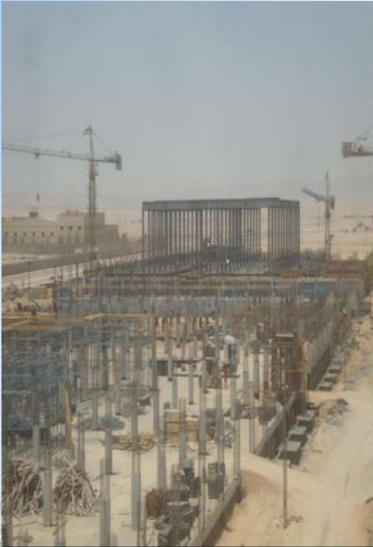
Workshops under construction
