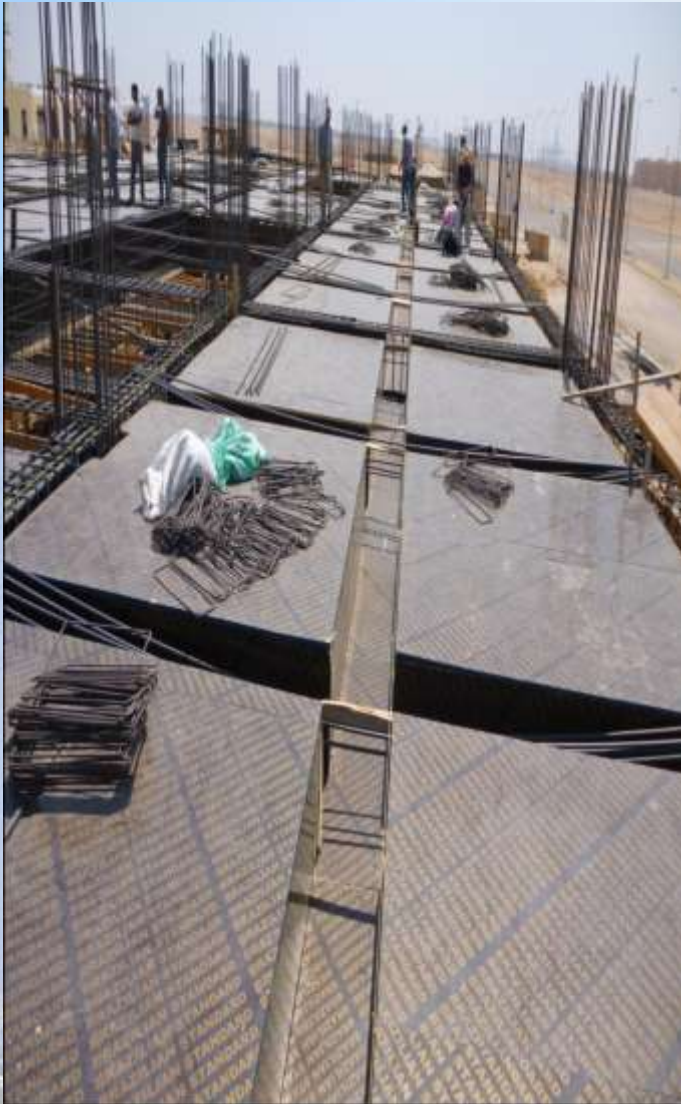
Construction of the fabrication area
