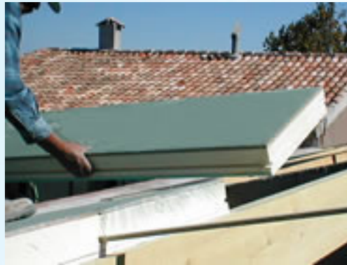
Roof insulation
