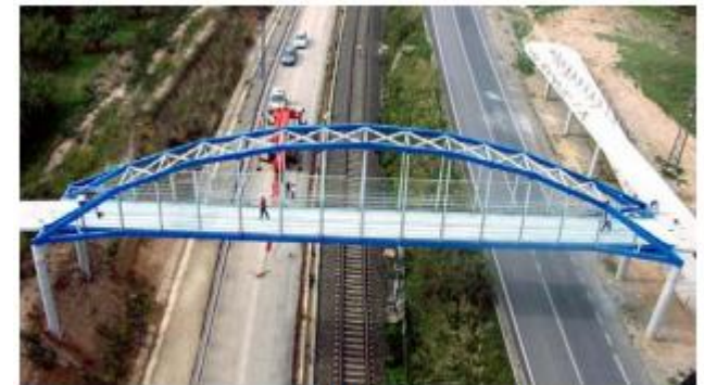
Fig.2. 38m span Lleida Footbridge, Spain (Fiberline).
