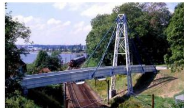
Fig.1. 40m long Fiberline Bridge, Kolding, Denmark.
